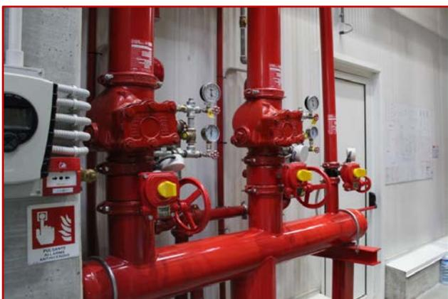
In addition to the typical automation systems, Cassioli supplied Sammontana also with an innovative fire-fighting system with related tank and water reserve that feeds it: specifically, a sprinkler system with internal and external hydrant network, pumping station and smoke detection systems, according to the current regulations.
